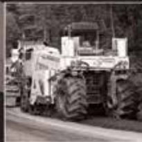
Full Depth Reclamation
