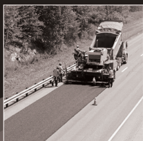
Paver Placed Surface Treatment
